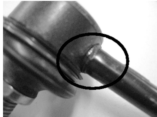
Fig. 7 Weld location on sway bar link
